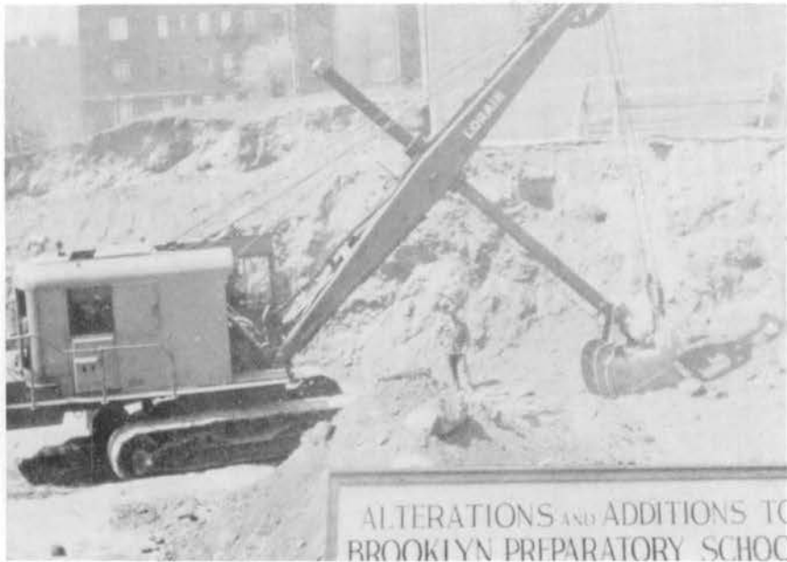
Construction begins on the new wing.
