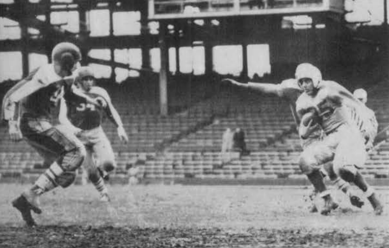
Mike Heaney looking for a hole.
